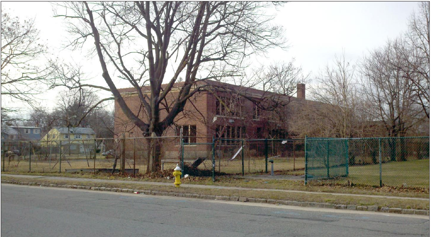
Site CC: Former Grand Street School; rear view looking northwest from Broadway
