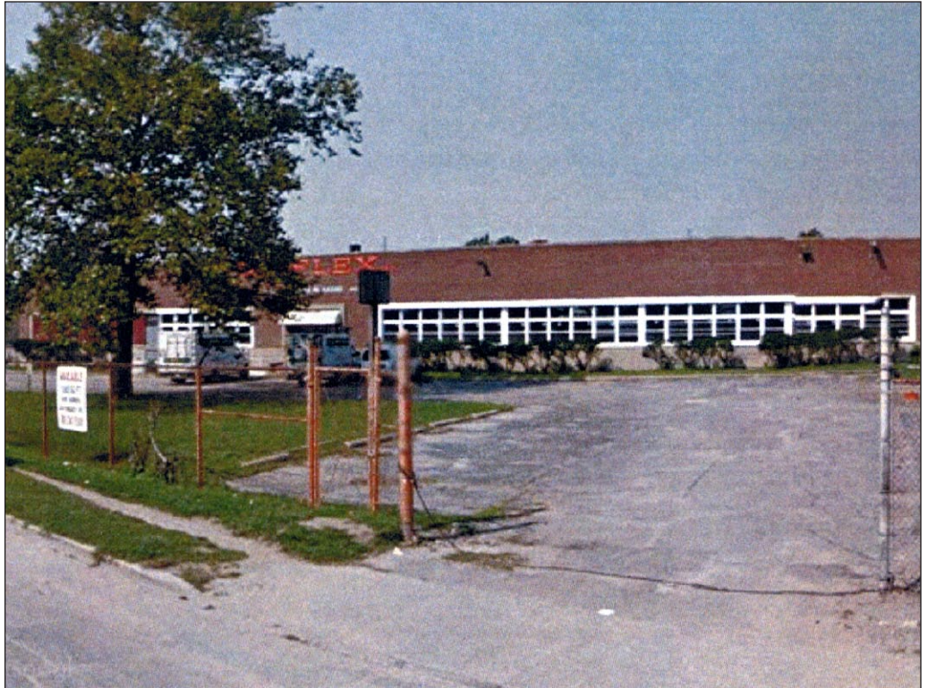
Site EE: Vacant Industrial/Warehouse Building, view looking northwest from Grand Boulevard 18
