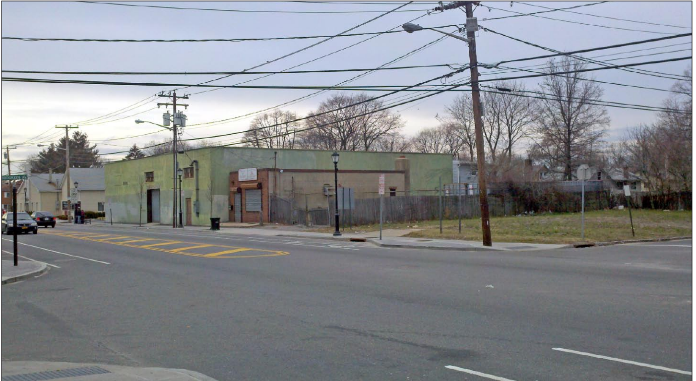
Site M: Vacant structure and adjacent lots; view looking northwest from Prospect Avenue 5
