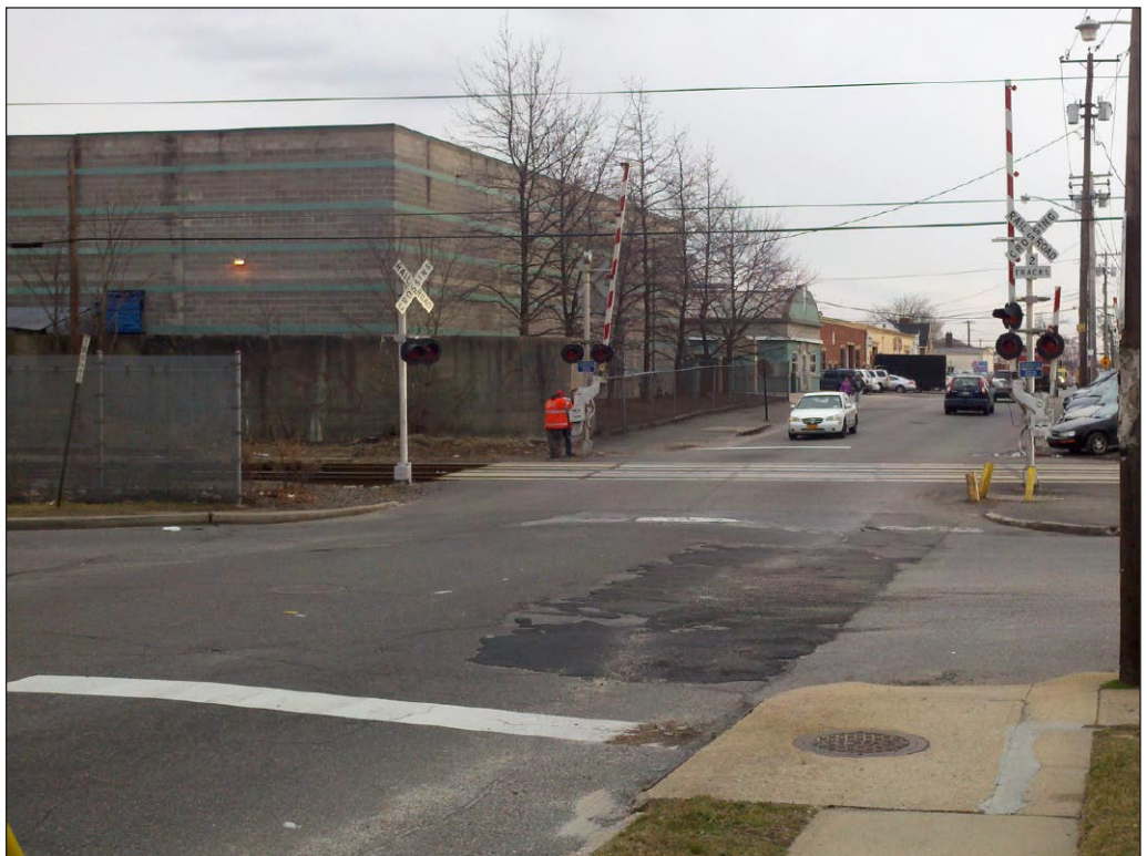
Site DD: LIRR Grade Crossing at Urban Avenue; view looking southeast from corner of Railroad Avenue and Urban Avenue 14
